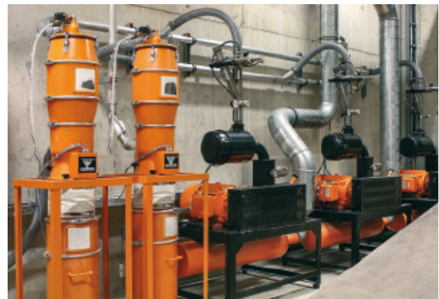
11 kW vacuum pumps with Sa 3 safety filters with 60 litre collection container
